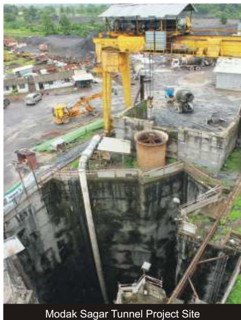
Modak Sagar Tunnel Project Site
